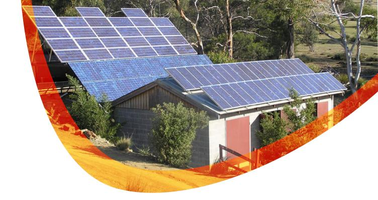
**Sunlight and panel placement** - Assess sunlight availability, considering shading from structures or trees and your area's climate. Our specialists will identify the best location, orientation, and tilt for solar panels to optimise efficiency. If your roof is small, consider a free-standing array, though it may increase costs.
