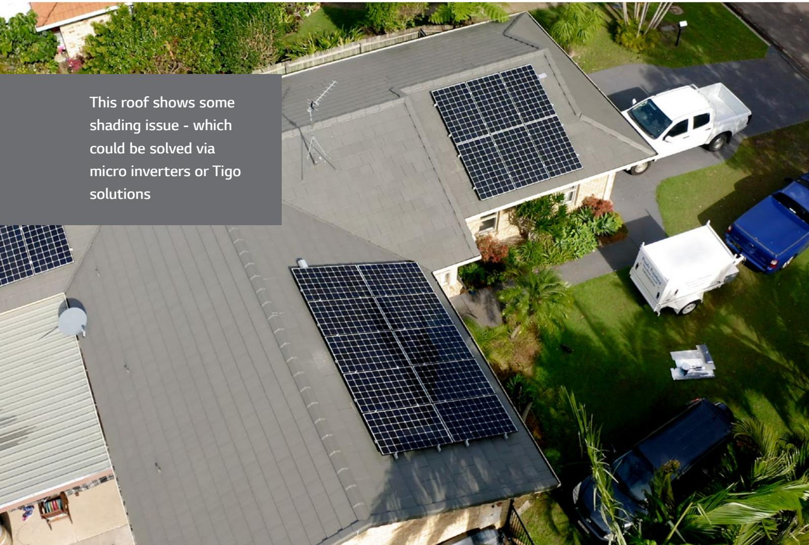
This roof shows some shading issue - which could be solved via micro inverters or Tigo solutions
